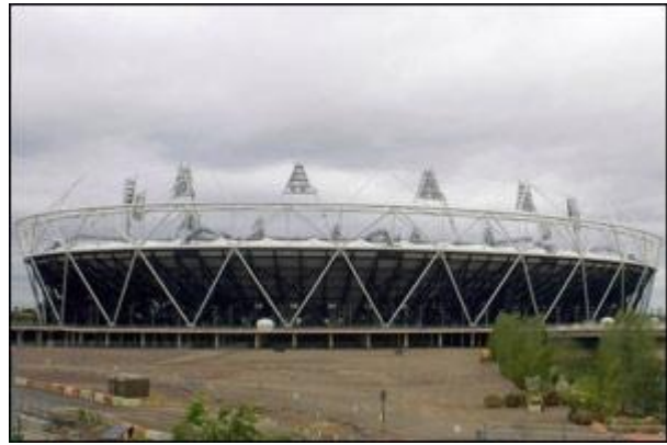
Construction is now complete at all six of the main Olympic venues
